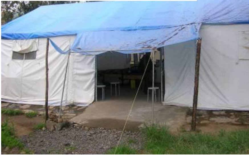
Gondar, Clinical Trial Center before rehabilitation
